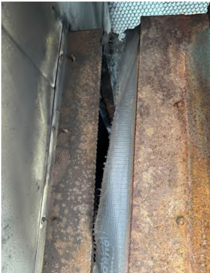
Inside Unit Separation between units
