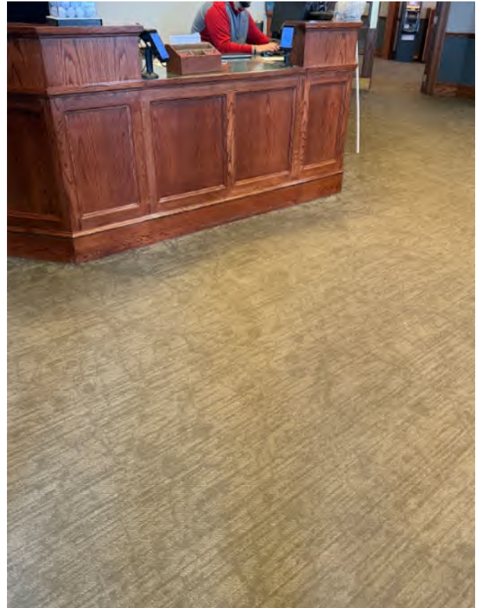
Pro Shop Wear pattern in same walking pattern and dirty in front of desk
