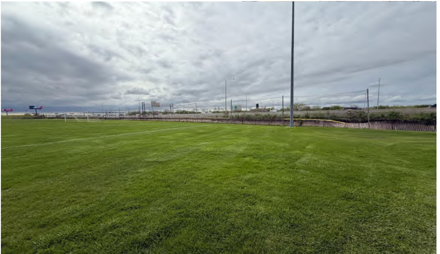
South soccer field netting and snow fence system
