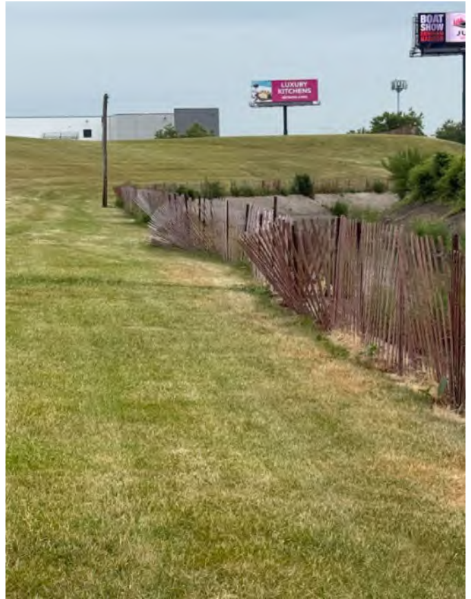
Snow fencing falling down
