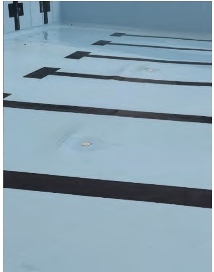
PEM matting shifting at existing inlets
